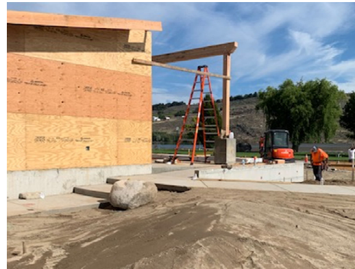
(Above) Setting grades (Below) Setting timbers for stage
