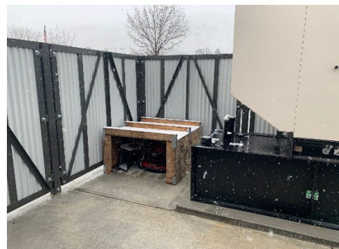
Dog house for lawnmower, so we are not keeping fuel in the pump station
